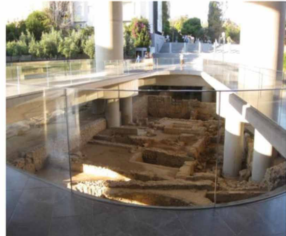
Fig. 2 The building located above Acropolis ruins
