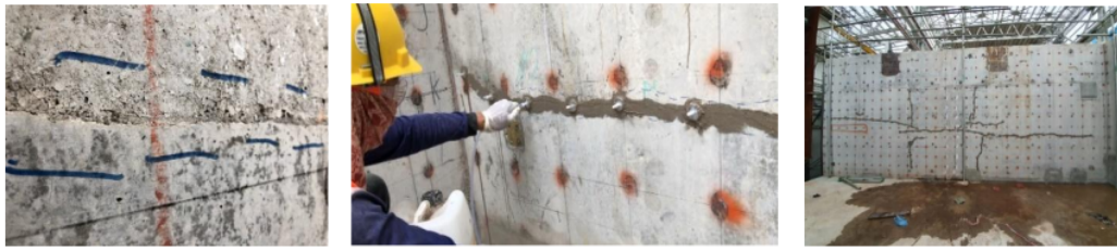
Figure 5. Repair work cold joint and cracks
