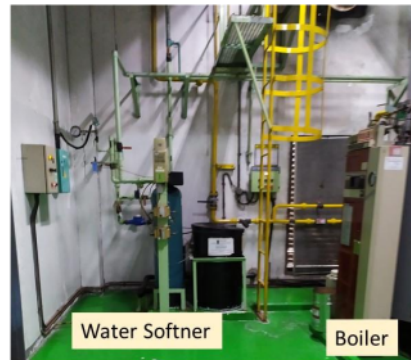
Figure 1. Boiler and Softner Layout
